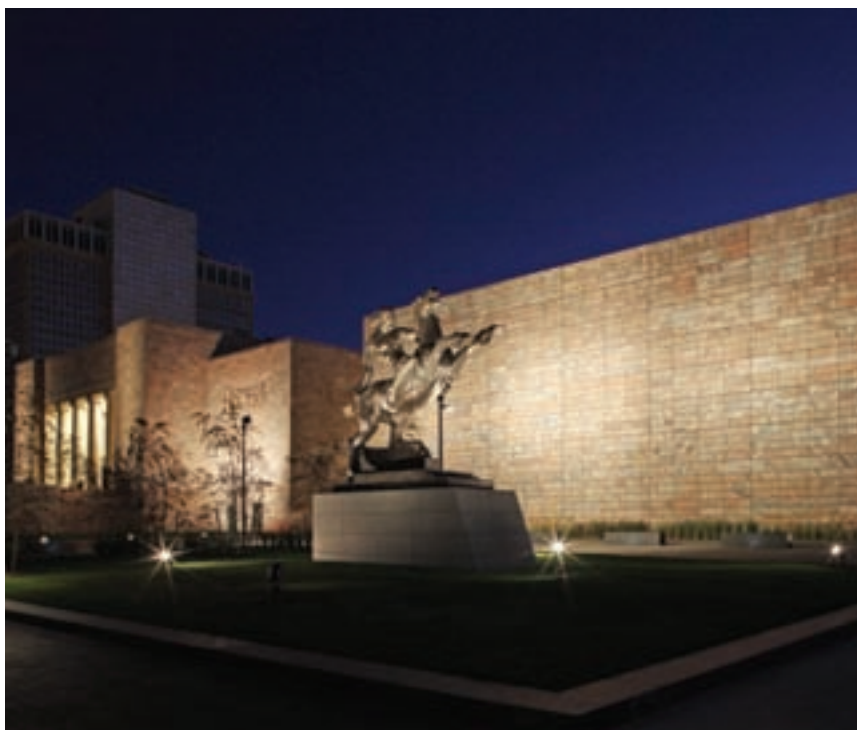
Limited set back necessitated different luminaires for façade lighting of the 1994 addition. The same CMH lamps were used throughout for color consistency. Sioux Warrior —a statue 70 years in the making—sits in front of the newly lighted façade.
