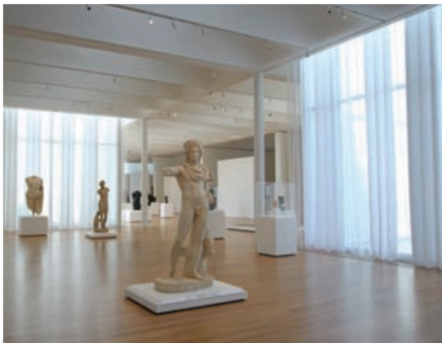
A combination curtain/roller-shade system controls sunlight entering the gallery space. Another control system operates the tungsten halogen track lighting mounted to spines between the ceiling coffers.
