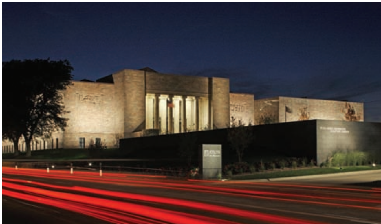
Illuminated for the first time, the pink marble façade of the 1931 museum building glows under 3,000K CMH lighting. Ground-mounted 150-W floodlights evenly wash the monolithic façade, while 70-W spots give extra punch to bas-relief friezes that depict the history of the American west.
